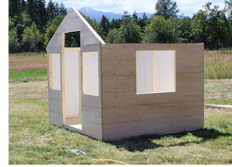
Wall assembly and front gable installed
