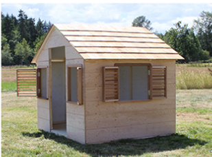
Install the windows and shutters
