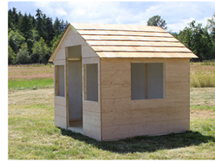
When both panels are in place, fasten them to the rafters using the finishing nails
