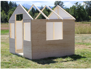
Join the rafters and set them evenly on the side walls
