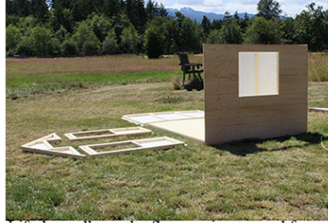
Lift the walls on the floor perimeter and fasten them together
